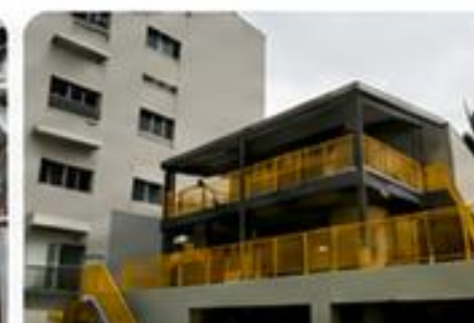
Wastewater Treatment Facility
